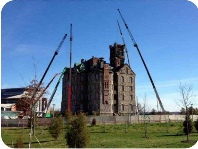
of the tower was saved in this way, along with a significant portion of the remainder of the building. The deconstruction and demolition team consisted of a crew of 17 masons, 13 environmental professionals, 15 demolition specialists, 2 engineers, and 4 full-time safety officers working together to create a successful project.
